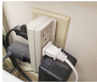
Adapter Flange Interferes
