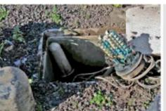
The orange 3/4-inch cable TV cable conduit was sitached to the 1-inch PVC conduit I had installed a foot underground some 5 years ago, planning ahead for possible cable TV installation without the need to break up concrete near my home.
