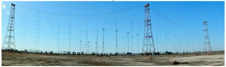
Two of five dipole curtain arrays at the VOA Delano Relay Site. Two others are visible in the background. The three towers are three hundred feet in height. Those in the background reach to four hundred feet!
