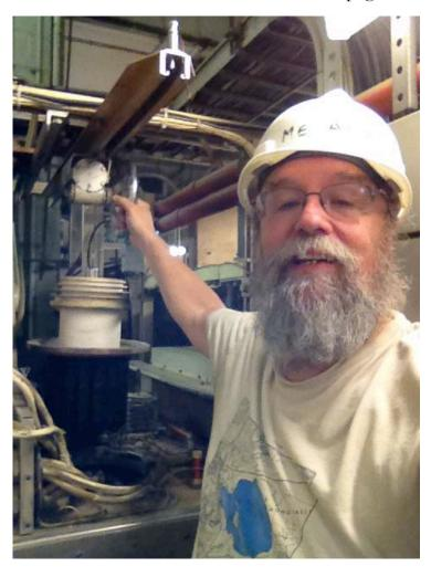
W6DQ gleefully removing one of four Eimac 4CV100000C vapor-cooled tetrodes from the PA compartment of transmitter DL-8. That is a 97 pound tube! Call it a case of "QRO envy!"
