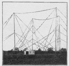
On the right is shown one of the earlier "wireless" stations. The vibrations of the waves from the sending instrument are carried up into the air on these wires and go out from them in all directions. Incoming waves are caught by the wires and carried down to the receiving instrument.
