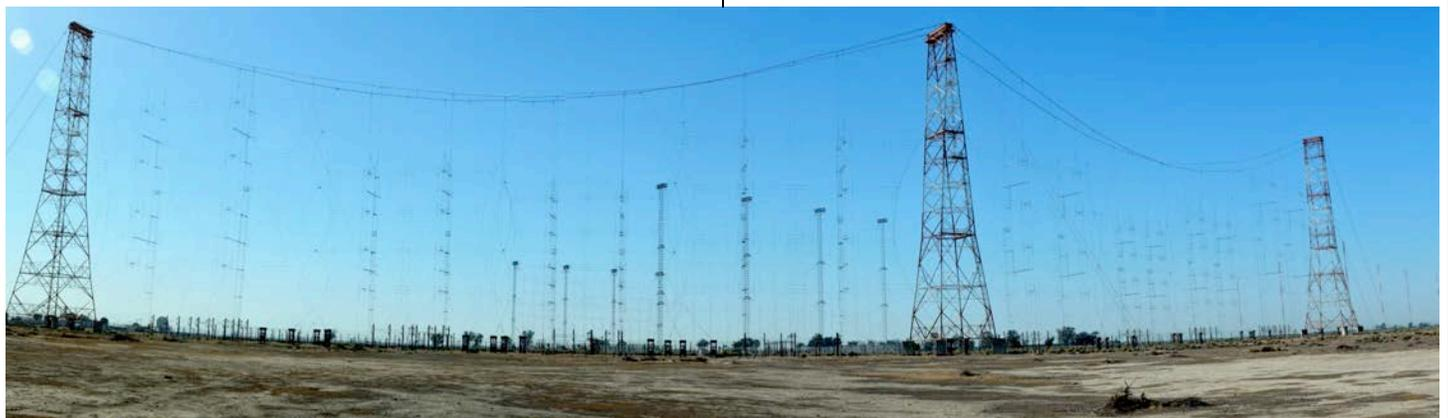
Two of five dipole curtain arrays at the VOA Delano Relay Site. Two others are visible in the background. The three towers are three hundred feet in height. Those in the background reach to four hundred feet!
